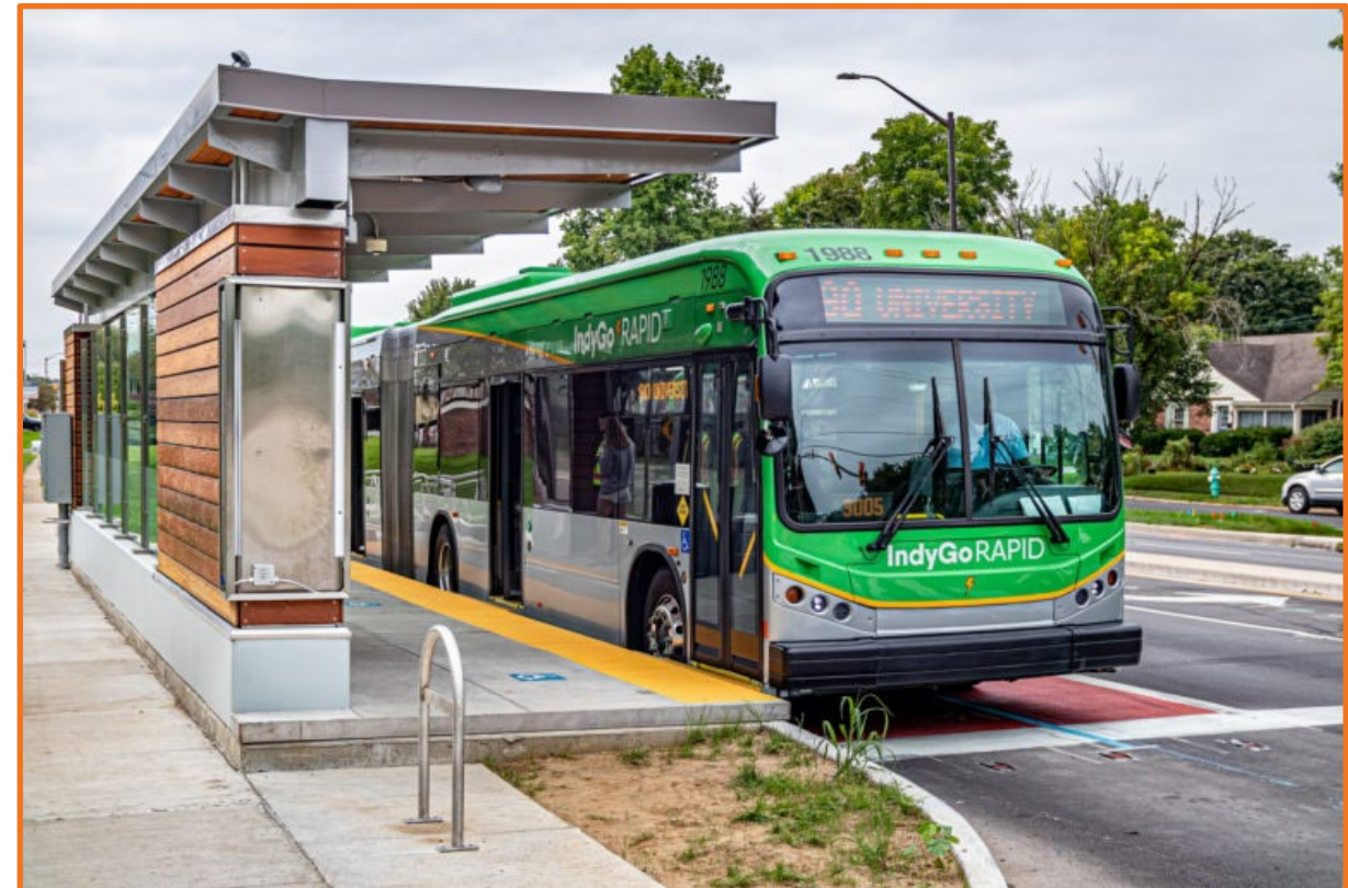
Red Line BRT in Indianapolis, IN
